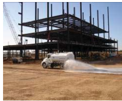
Construction Parking Parking Lot Dust Control Haul Road Dust Control Parking Lot Solidification
