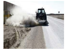
Road Shoulders Shoulder Dust Control Shoulder Erosion Control Shoulder Stabilization
