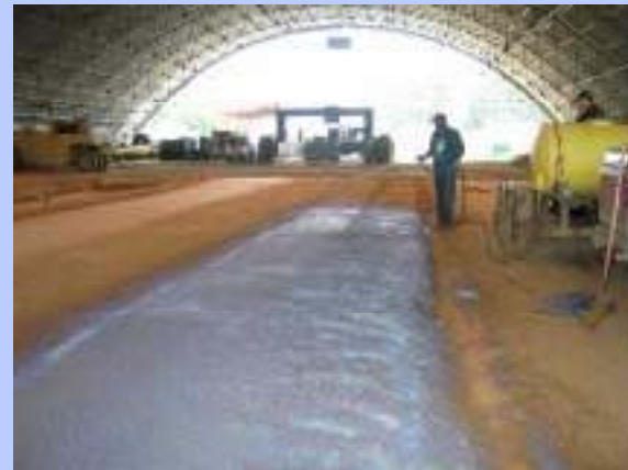
Added the Stabilizer
