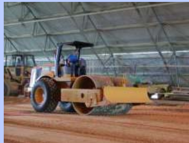
Compacted to 95% Proctor
